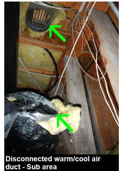
Disconnected warm/cool air ducts - Attic
