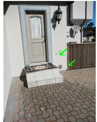
Hand railing is recommended for safety
