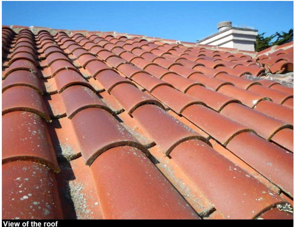
View of the roof
