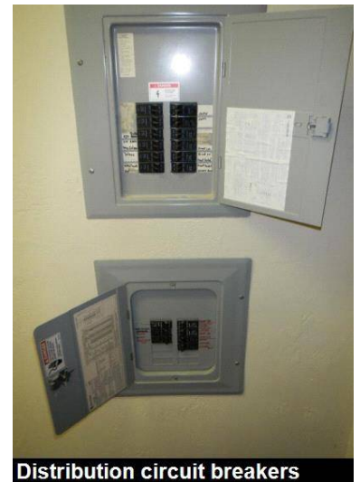
Distribution circuit breakers
