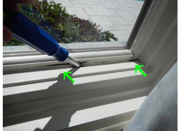
Damaged wood window frame - Kitchen
