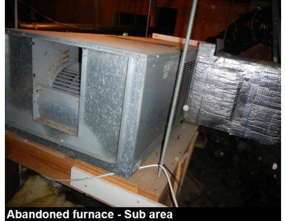
Abandoned furnace - Sub area
